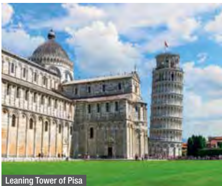
Leaning Tower of Pisa
